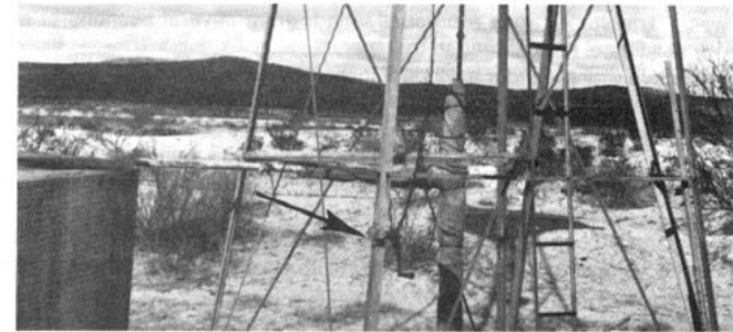
Windmill. Note windlass (arrow).
