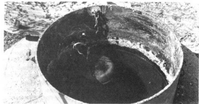
Float-valve regulates water level in stock tank.
